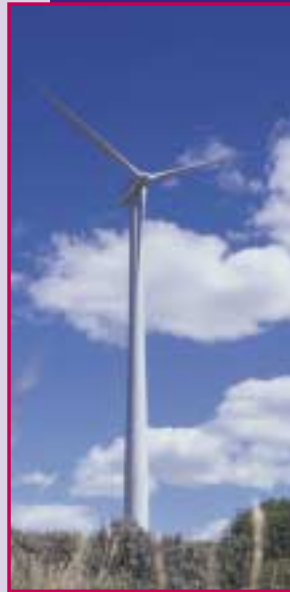
The first of 17 wind turbines at SunBridge installation near Gull Lake, Sask
